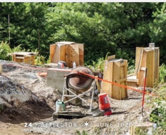
Summer 2014: it all starts with poured concrete piers. Plywood forms were shaped to fit the contours of the bedrock. Members mixed the concrete with the mixer in the foreground. Photo by Michael Patterson.
