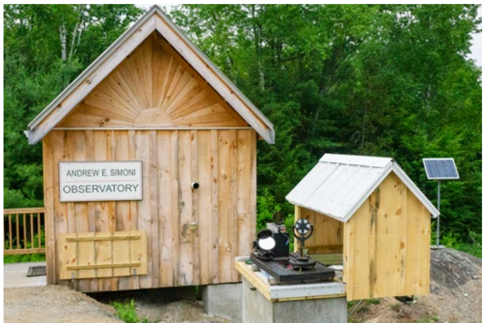
The Simoni Observatory houses the spectroheliometer at Stellafane. The roll-off "doghouse" in the foreground shelters the coelostat and objective singlet on their concrete pier. Light enters the building through the small tube protruding from the wall; the scanning prisms, slits, diffraction grating, and collimating and focusing mirrors are mounted inside on two concrete piers anchored in the bedrock below. The entire observatory is powered by batteries charged by the small solar panel in the background. Photo by Michael Patterson.
